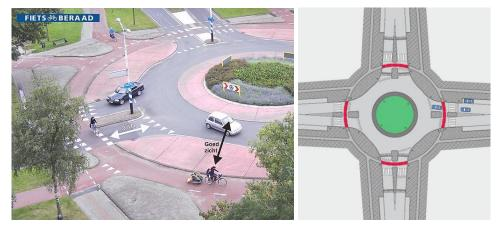
Single-lane roundabout with cycle track, with right of way for cyclists (Enschede, NL). Notice the typical circular design of the track and the colored crossings.
